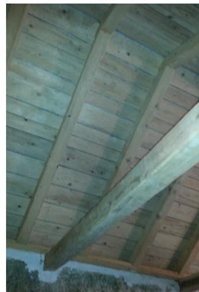
75. Obnovljeni krov – A restored roof – Erneuertes Dach
