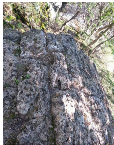
90. Sedreni krov odozgo – Tufa roof from above – Travertin-Dach von oben
