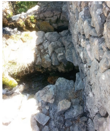
57. Jaža na ulasku u Gužvica mlin – A sluice at the entrance to the Gužvica watermill – Mühlgraben am Eingang in die Gužvica-Mühle
