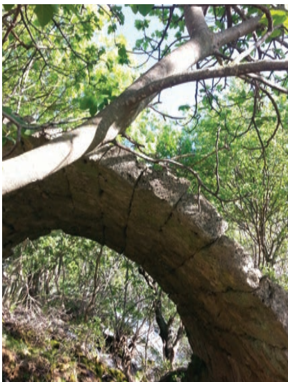
84. „Ćemereni“ sedreni krov mlina – A traditionally – built tufa roof of the watermill – Travertin-Dach der Mühle
